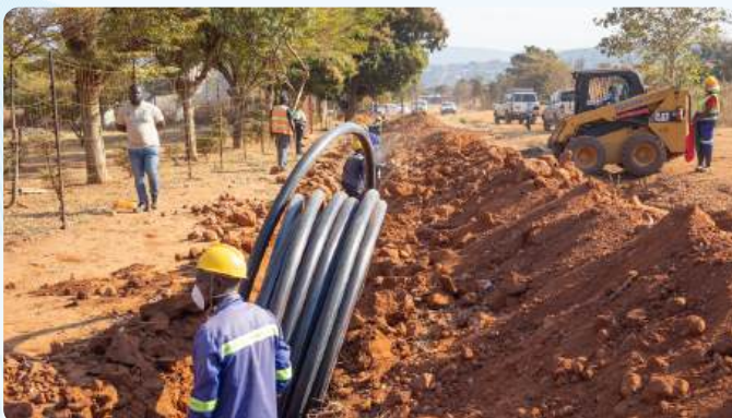
Worker pauses for the PS - MWDS Eng. Romas Kamanga as he tours the project
